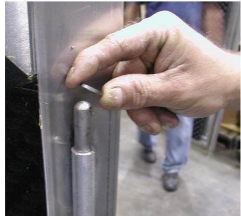
6. Position one person inside and one outside. Remove 1/2-13 x 7" bolts, nuts and washers that fasten the panels together. There may be silicone caulk between the roof and top of the panels.
