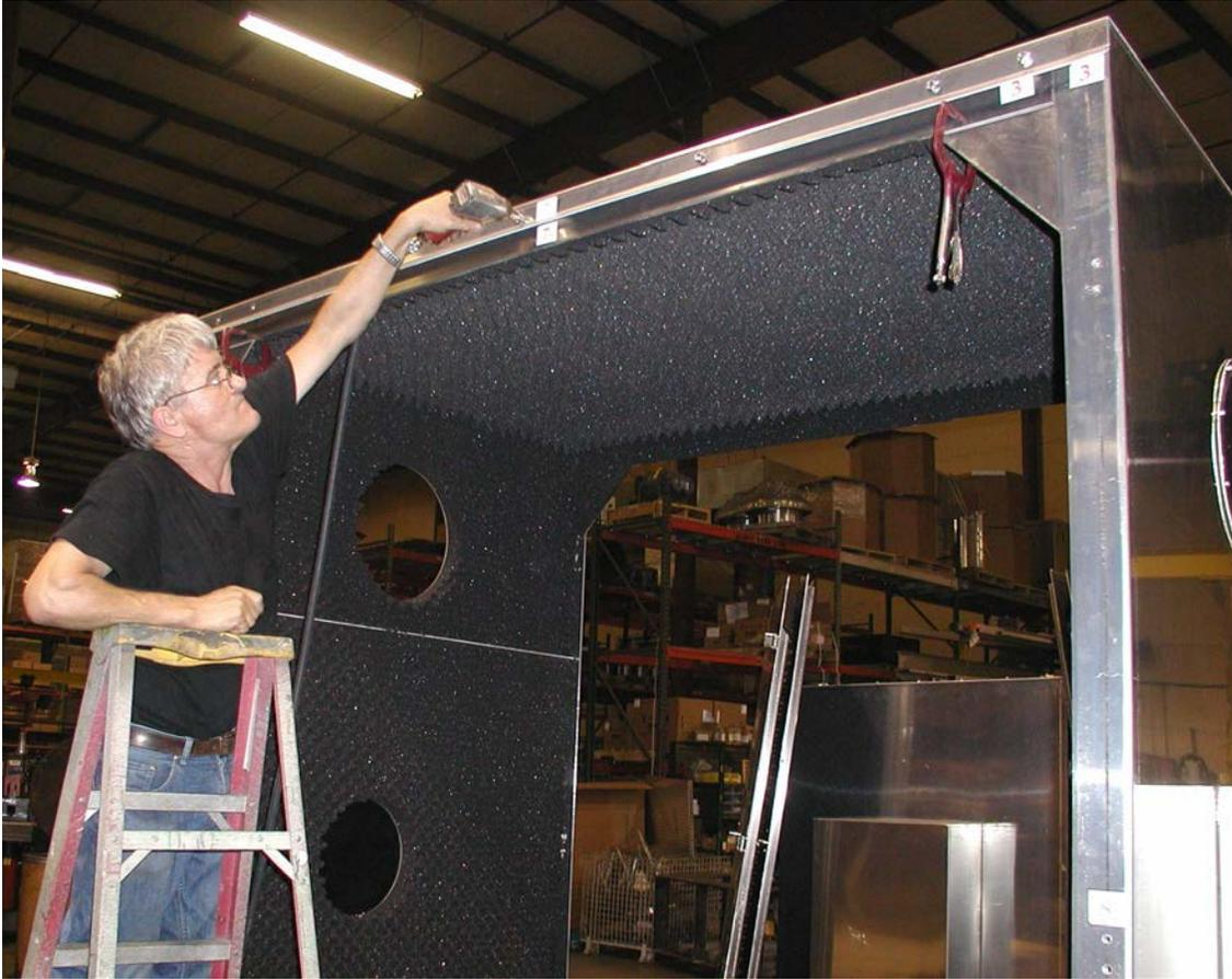
11. Use 3/8 Bolts to fasten the Roof Panel to the End Panels.
