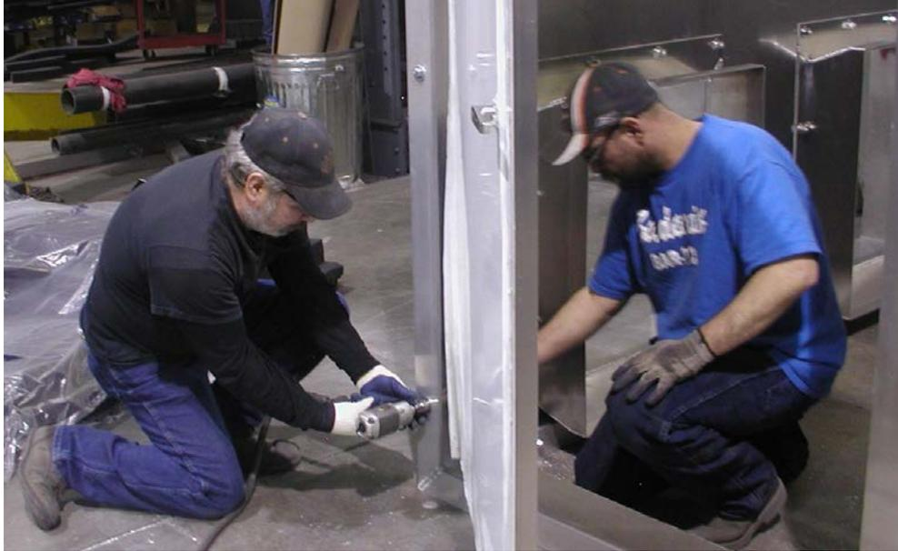
3. Locate the next wall panel. Stand upright. If provided, use silicone caulk between the panels.
